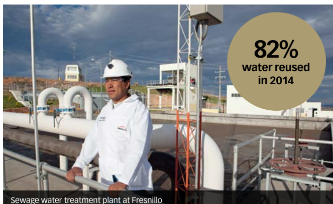
Sewage water treatment plant at Fresnillo
