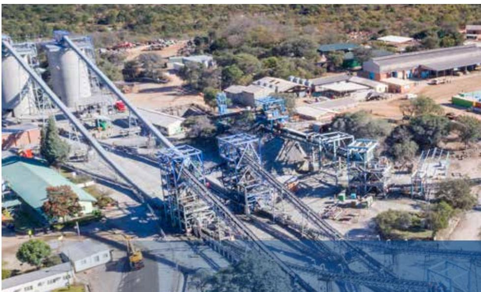
MIMOSA IS JOINTLY HELD BY IMPLATS AND SIBANYE-STILLWATER. ITS OPERATIONS ARE LOCATED ON THE WEDZA GEOLOGICAL COMPLEX ON THE ZIMBABWEAN GREAT DYKE, 150 KILOMETRES EAST OF BULAWAYO. THE OPERATION COMPRISES A SHALLOW UNDERGROUND MINE, ACCESSED BY A DECLINE SHAFT, AND A CONCENTRATOR.
