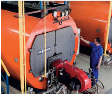
Belvedere: R&D to install a biomass-fueled power plant.
