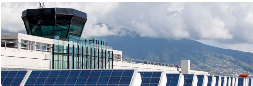
Solar panels installed at La Palma Airport.
