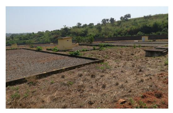
**Photo 28.** Sewage treatment works, Sangaredi. Vegetation removed from filter beds.
