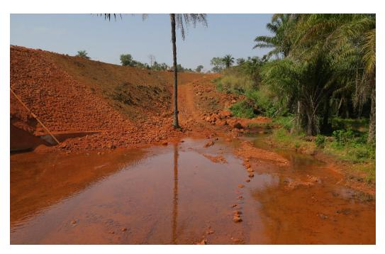
Photo 34. Thiapikour river crossing – poor erosion control/evidence of sedimentation
