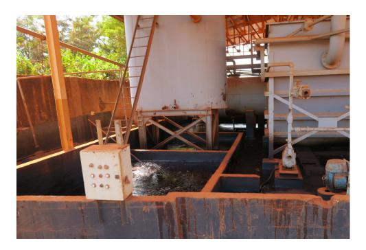
**Photo 18.** Heavy oil contamination at decommissioned oil water seperator
