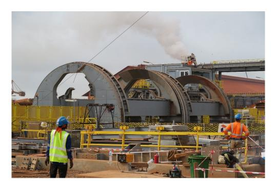
**Photo 1.** Newly constructed dual wagon tippler
