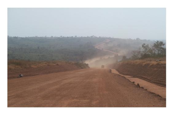
Photo 35. Limited evidence of dust control on COBAD Road
