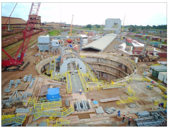
Crusher pit and tippler in foreground, ramp and secondary sizer in the background. Conveyor to existing plant visible.
