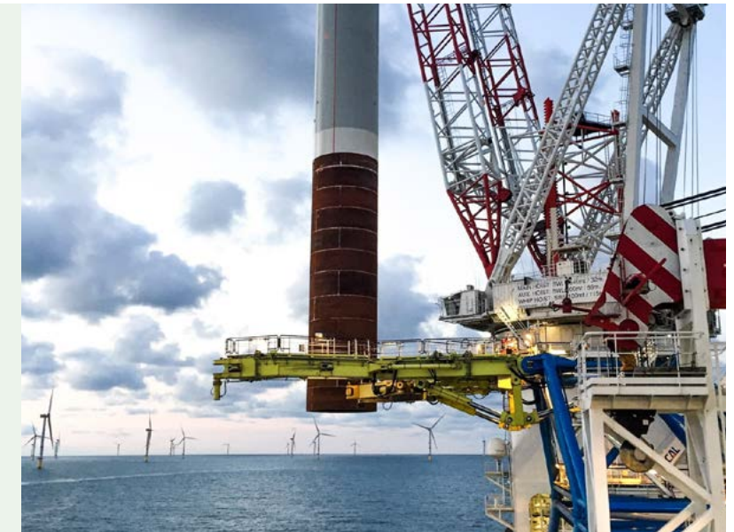
Northland Power's Deutsche Bucht wind farm (under construction).
