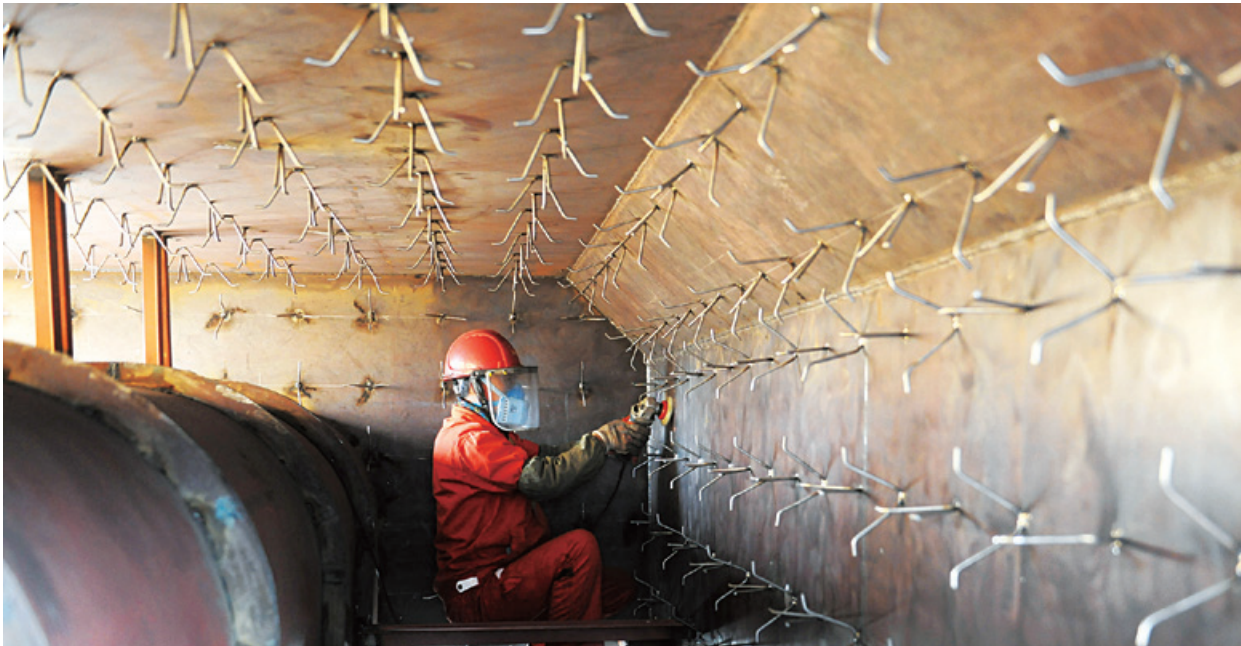
▲ PetroChina Jinzhou Petrochemical Company makes every effort to ensure operational safety
