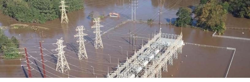
Duke Energy electrical substation immersed in floodwaters after Hurricane Florence.
