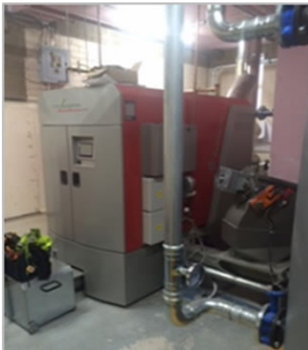
Biomass boiler in PMUK
