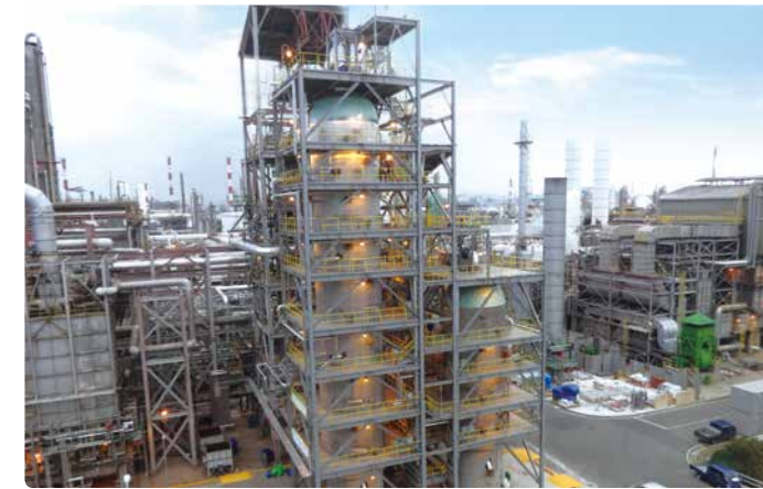
Completed the upgrade of the hydrocracker
