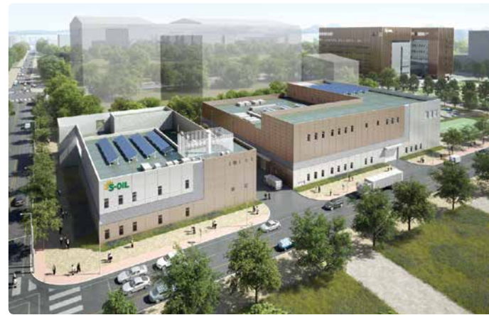
Fuel Oil/Lube Oil Engine Test Building and Chemical TS Center (Bird's-eye View)
