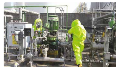
Shutoff of leakage source
