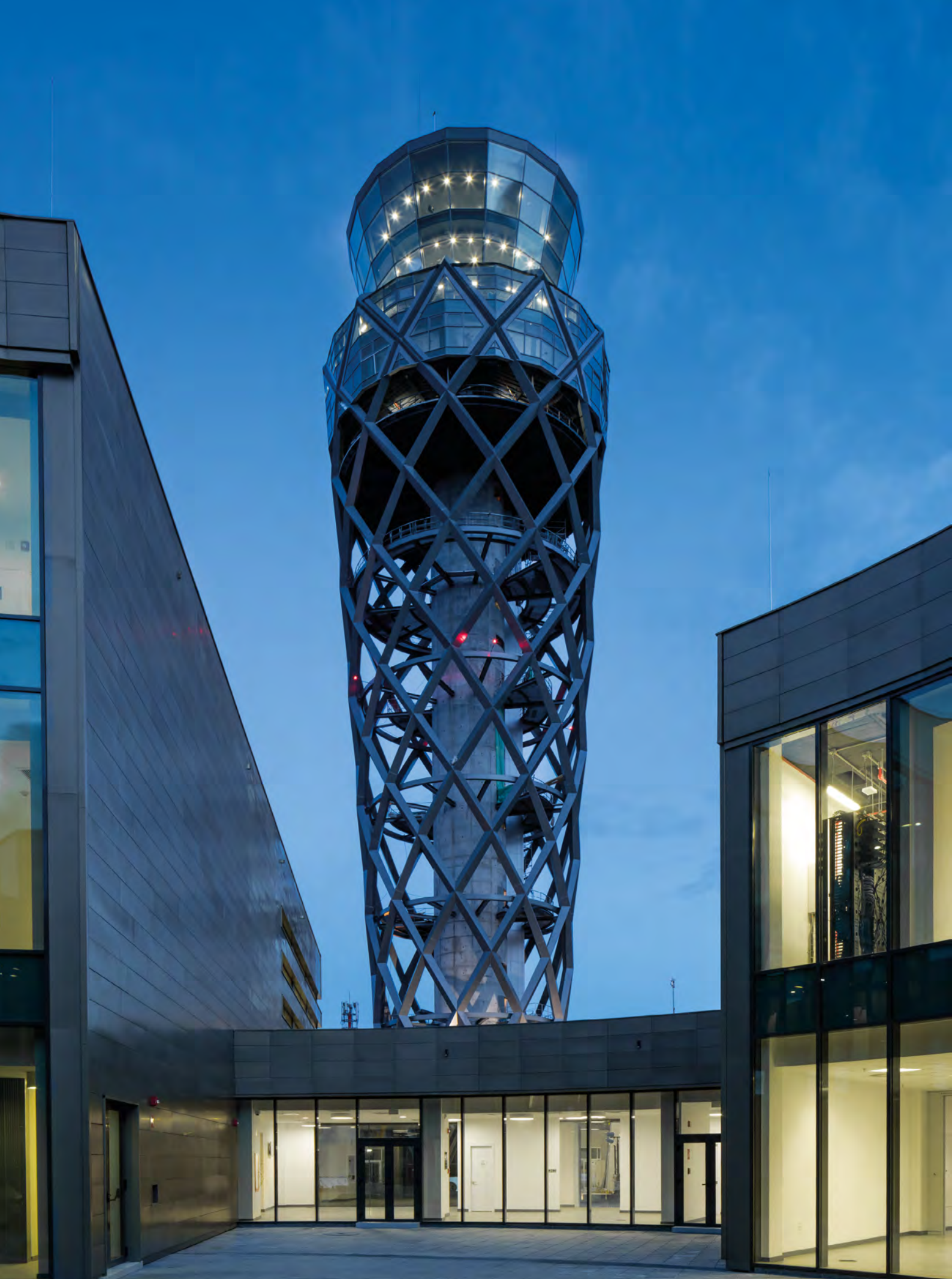
Control tower of El Dorado's airport, Colombia
