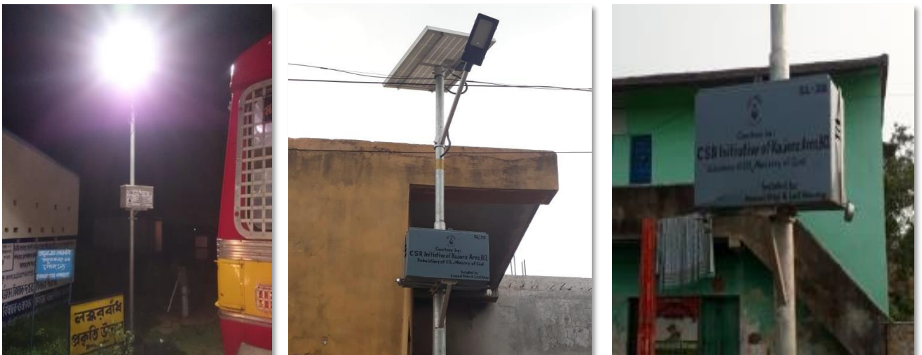
Fig. - Installed streetlights in 127 villages in West Bengal's Paschim Bardhaman District
