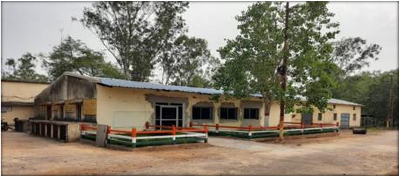
Fig. - Exterior View of under-construction museum
