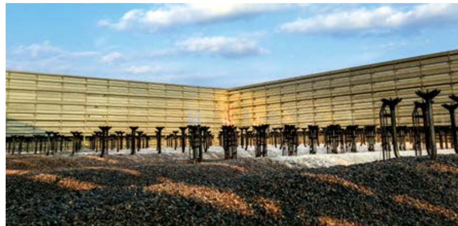
📍 Sino-Korean Petrochemical uses ground-based high-pressure flares and drone monitoring to reduce methane emissions
