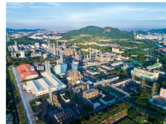
Guangzhou Petrochemical facilities covered in green
