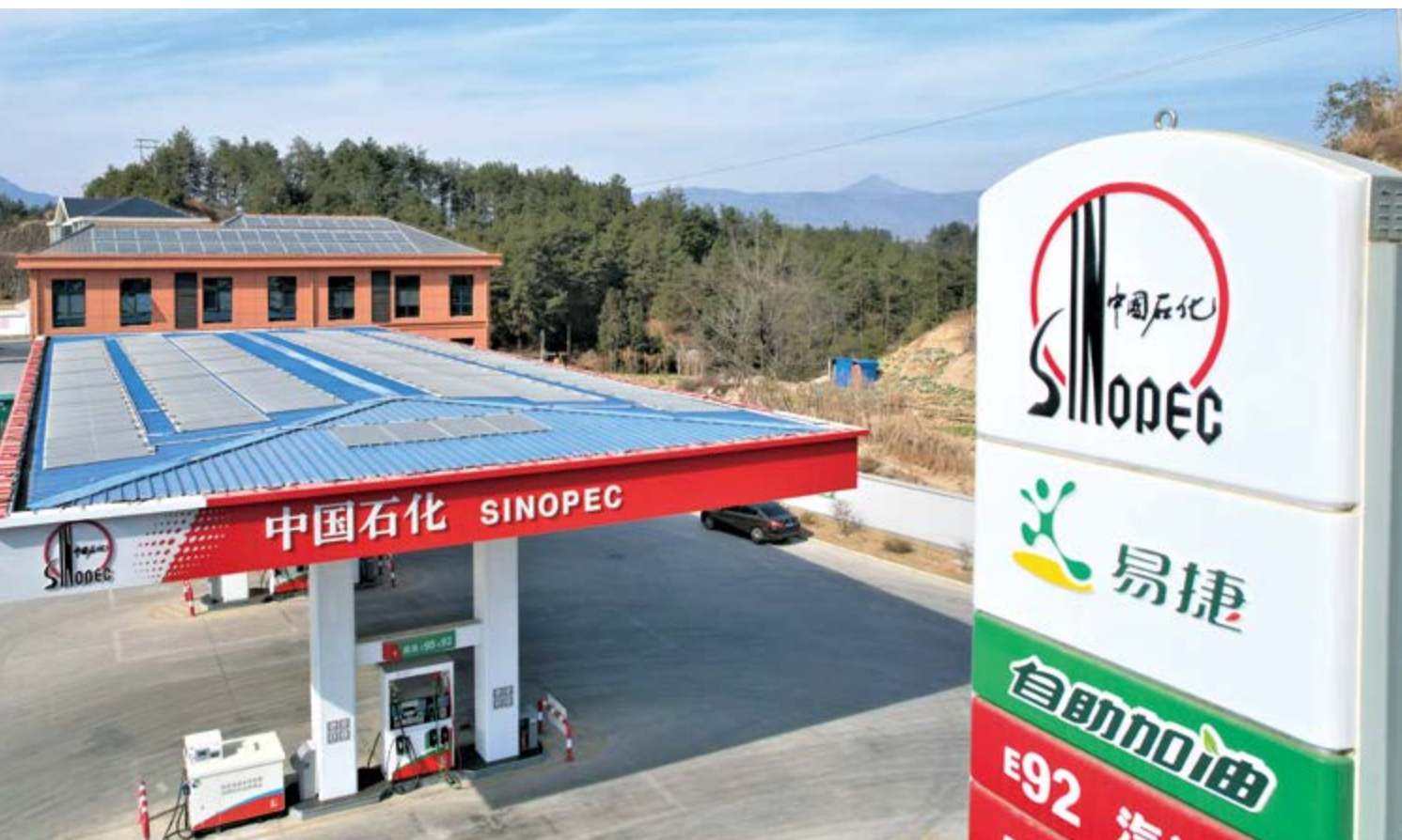
Ⓐ Rooftop photovoltaic power generation unit at Jiaze refuelling station in Changzhou, Jiangsu generates 127,000 to 147,000 kWh of electricity annually
