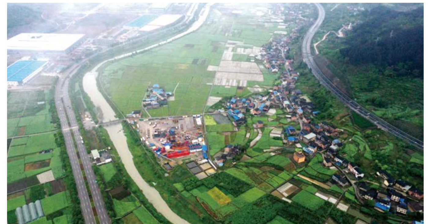
Ⓐ Huadong Petroleum Engineering Company's Shengye 2 platform minimises land use during the construction process
