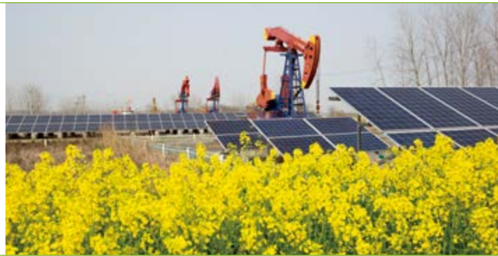
④ Jiangsu Oilfield powers the pumping unit with photovoltaic power
