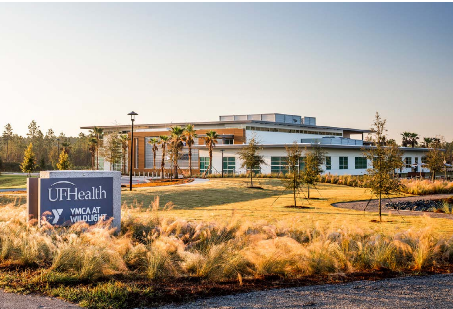
Yulee Medical Office Building | Yulee, FL
