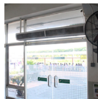
Air curtains for preventing entry by insects
