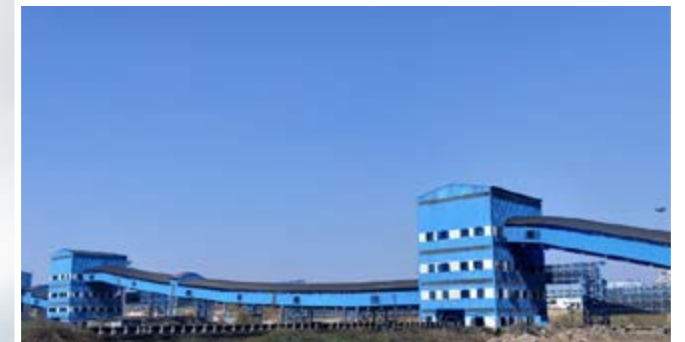
CHP NTPC Darlipali – 2X800 MW
