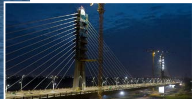
Karimnagar Cable Stayed Bridge
