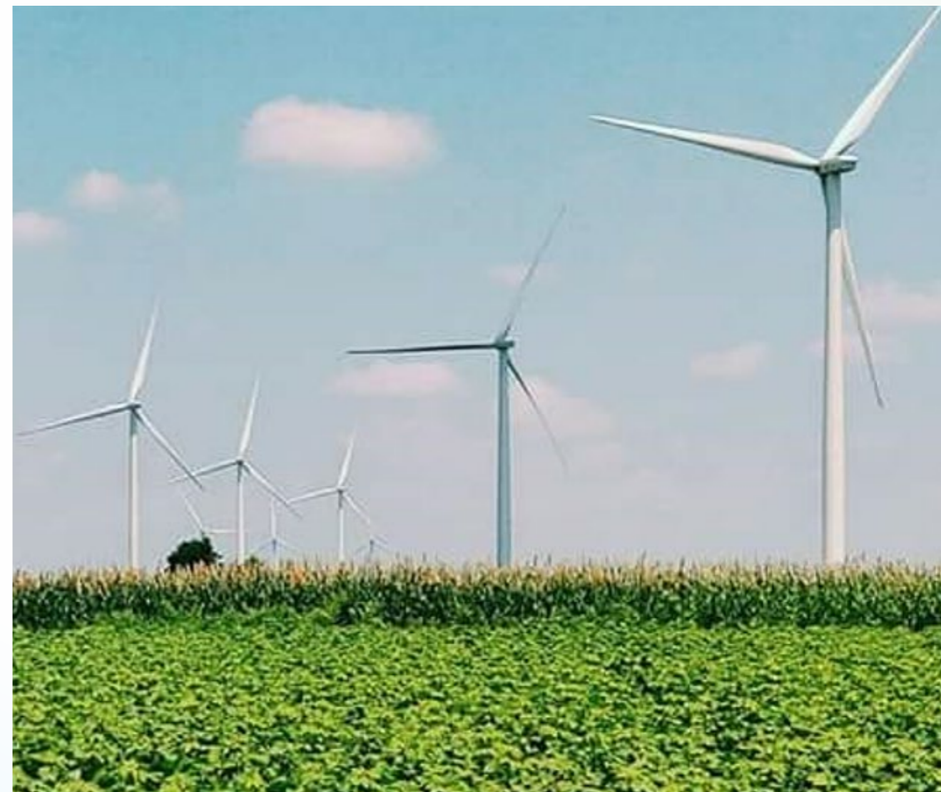
Windmills installed in Andhra Pradesh by a SBI financed group.
