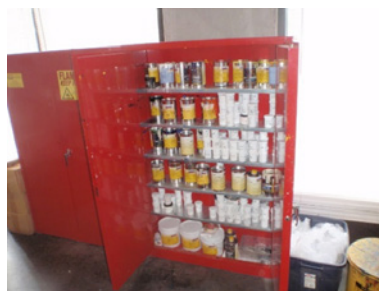
Proper storage of flammable liquids in a designated and properly designed cabinet.
