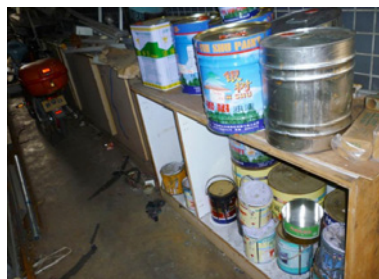
Poor storage of flammable liquids.
