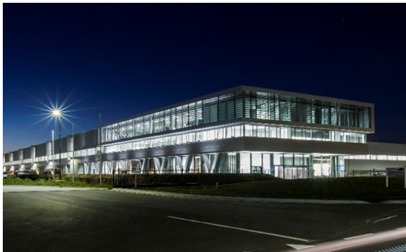
Venlo Distribution Center
