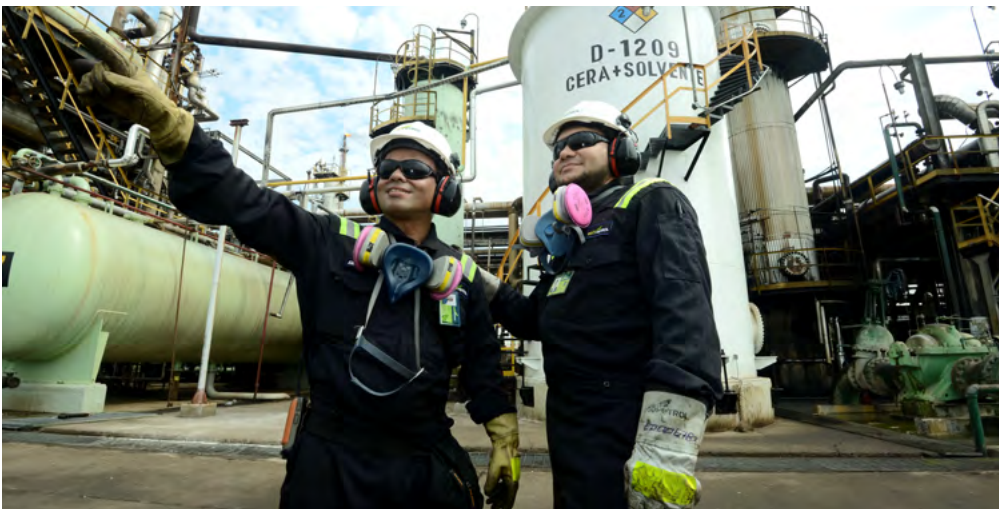
Paraffin unit, Barrancabermeja refinery
